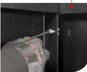
4. Using the bolts provided, insert and tighten using a 4mm Allen key. Ensure that the top edge of the planter is flush before tightening.
